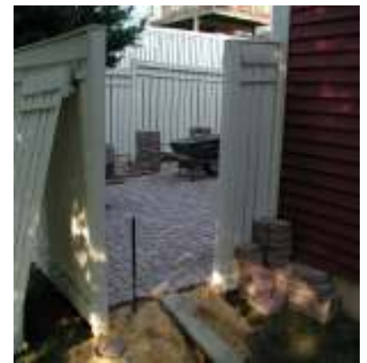
Patio during construction
